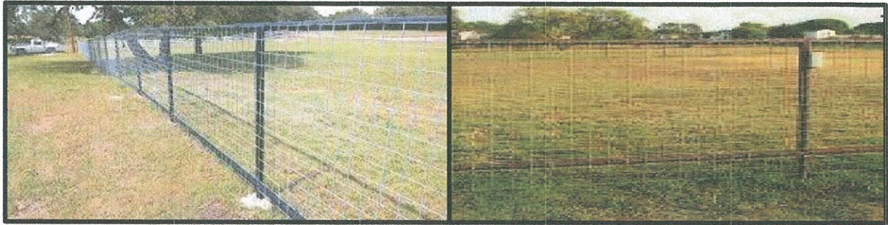
Steel pipe fence
